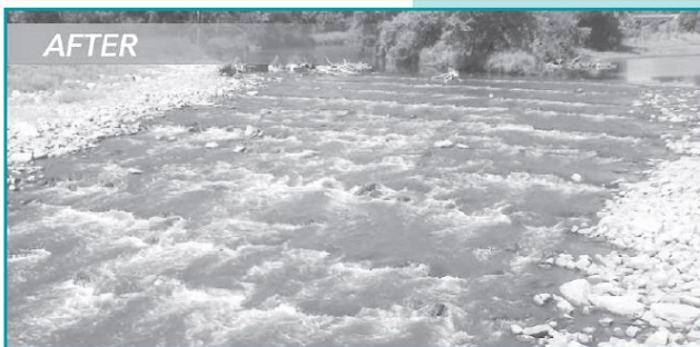
Klondike Mill Dam on the Big Sioux River, retrofitted to create rock arch rapids; photo by the Iowa Department of Natural Resources.
